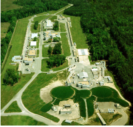
Figure 1.1: Aerial view of Jefferson Laboratory (JLAB) facing east. Image source: [23].
